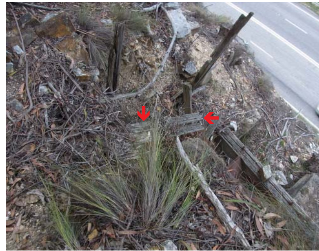
FIGURE 7.12: Looking at the input chute from the right side. The timber board (red arrows) was probably part of the floor of the chute. The chunks of chert would have tumbled down the chute into the crusher. (Oct. 2014)
