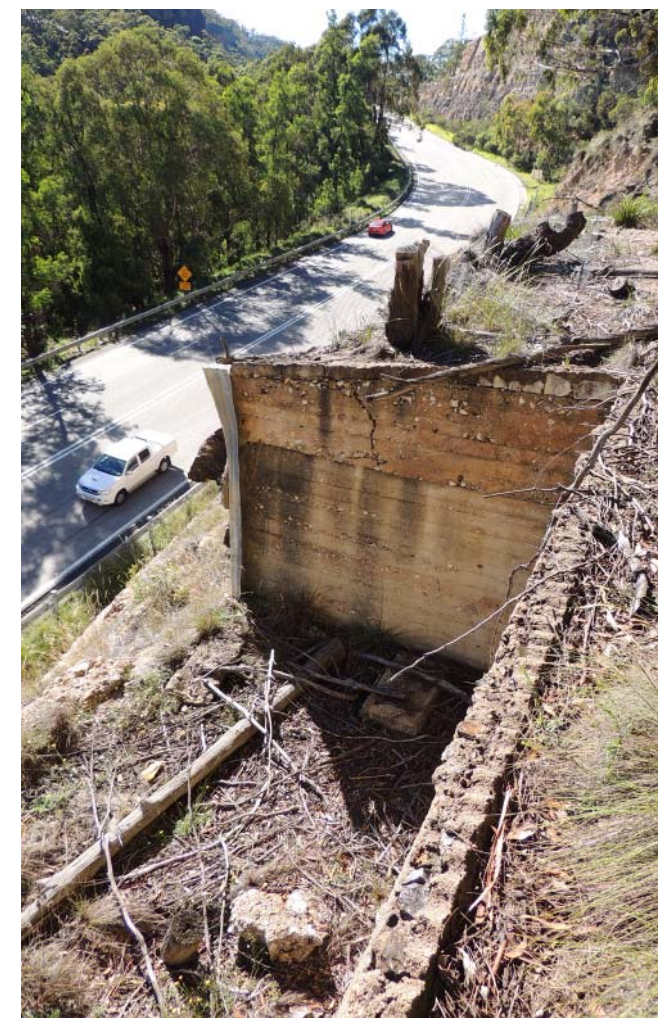
The two photos above and the one at bottom left show the concrete structure that housed the Jaques rock crusher. Top left — FIGURE 7.15: Looking down and east, from above. Note the concrete base for the motor in the right corner. (See photo at bottom right.) Top right — FIGURE 7.16: Photographed from within the structure looking east towards Mitchells Causeway. Note the timber beams and steel plates of the chute that was below the crusher. Also the bolts which secured the crusher to the beams. Bottom left — FIGURE 7.17: Looking west from within the structure. The jumble of timbers just beyond the steel chute were part of the chute into which chert was tipped to fall down into the crusher. The conveyor belt would have started below the steel plates and carried the crushed chert to the rotary screen for sizing and into the bins which would have been to the right and below. Photos by Brian Fox, January 2015.
