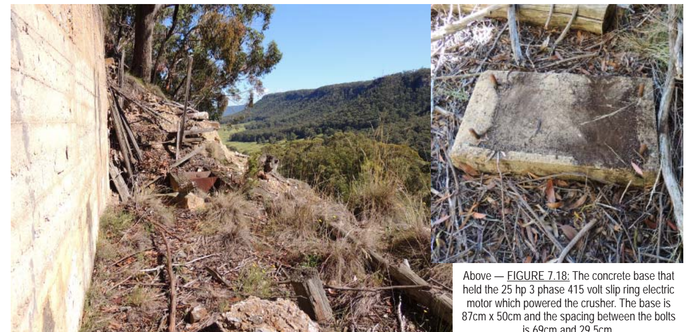
The two photos above and the one at bottom left show the concrete structure that housed the Jaques rock crusher. Top left — FIGURE 7.15: Looking down and east, from above. Note the concrete base for the motor in the right corner. (See photo at bottom right.) Top right — FIGURE 7.16: Photographed from within the structure looking east towards Mitchells Causeway. Note the timber beams and steel plates of the chute that was below the crusher. Also the bolts which secured the crusher to the beams. Bottom left — FIGURE 7.17: Looking west from within the structure. The jumble of timbers just beyond the steel chute were part of the chute into which chert was tipped to fall down into the crusher. The conveyor belt would have started below the steel plates and carried the crushed chert to the rotary screen for sizing and into the bins which would have been to the right and below. Photos by Brian Fox, January 2015.
