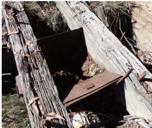
FIGURE 7.13: The two timber beams would have supported the crusher — see the bolts that secured the machine. The crushed stone fell between the steel plates through the angled steel chute onto the conveyor belt. Photo by Brian Fox, 2015.
