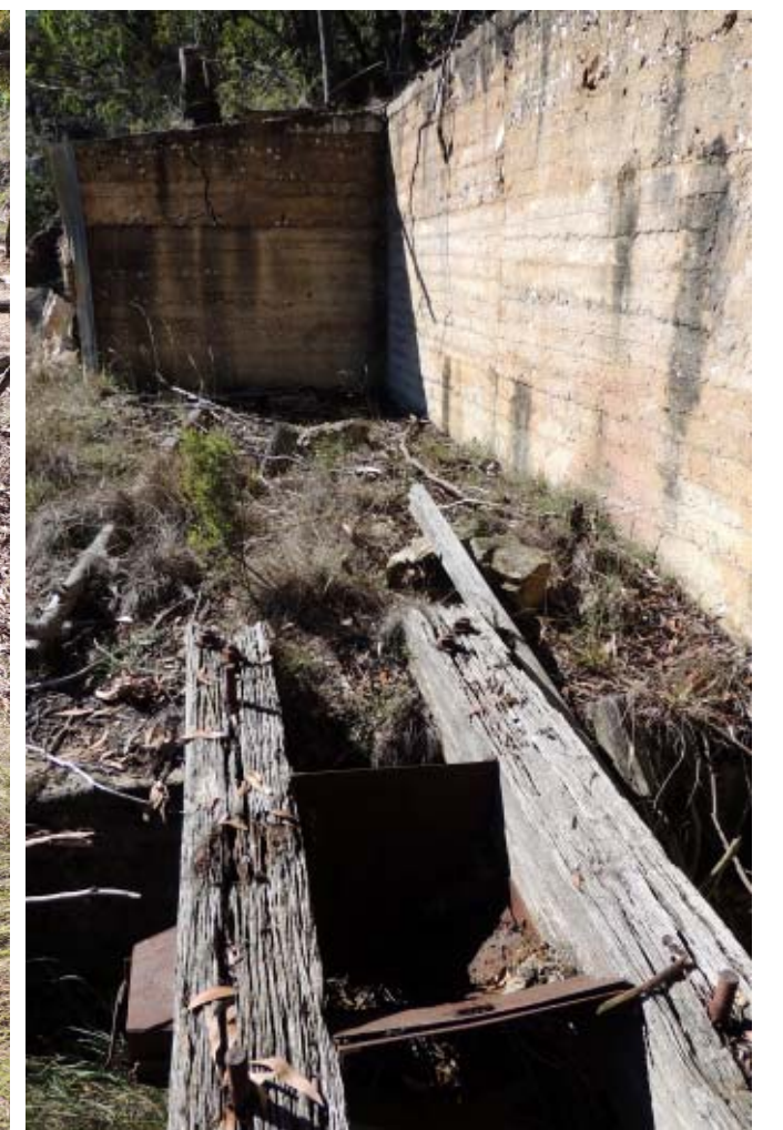
The two photos above and the one at bottom left show the concrete structure that housed the Jaques rock crusher. Top left — FIGURE 7.15: Looking down and east, from above. Note the concrete base for the motor in the right corner. (See photo at bottom right.) Top right — FIGURE 7.16: Photographed from within the structure looking east towards Mitchells Causeway. Note the timber beams and steel plates of the chute that was below the crusher. Also the bolts which secured the crusher to the beams. Bottom left — FIGURE 7.17: Looking west from within the structure. The jumble of timbers just beyond the steel chute were part of the chute into which chert was tipped to fall down into the crusher. The conveyor belt would have started below the steel plates and carried the crushed chert to the rotary screen for sizing and into the bins which would have been to the right and below. Photos by Brian Fox, January 2015.
