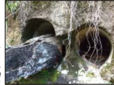
Trestle support timbers were cemented into holes gouged in the cliff.
