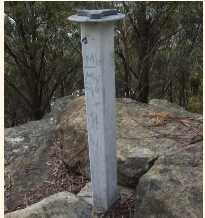
*Figure 6: Bracey Trig Station steel pillar.*
